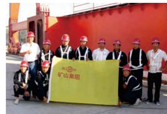
Our installation terms install 150t gantry crane in russia
